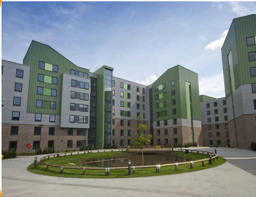
Completed project August 2011
